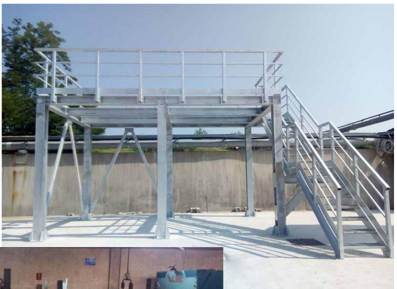
Balcony for aggregate processing plant
